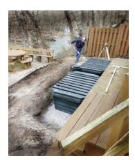
pad situated directly beneath the modules for dispersal into the native soil
