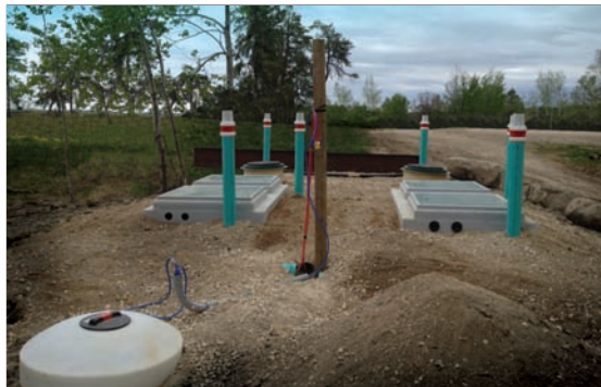
After installation of the two Platins
