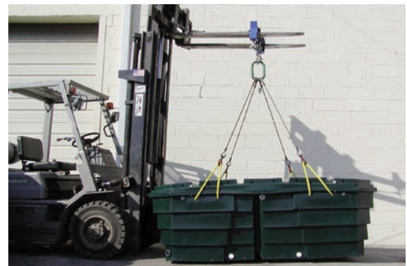
Figure 2 Module Off-loading
